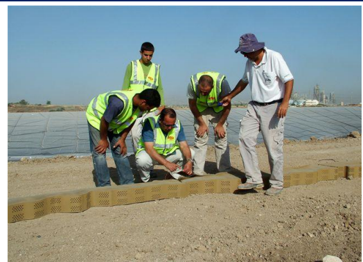
FIGURE 11. LAYOUT SECTIONS ALONG CREST SLOPE
