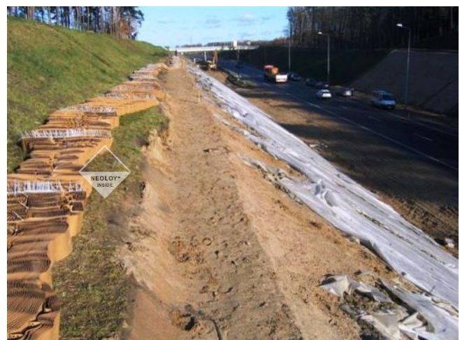
FIGURE 5. TRENCH ALONG SLOPE CREST
