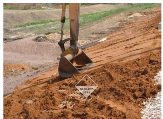
FIGURE 19. BLADE COMPACTION
