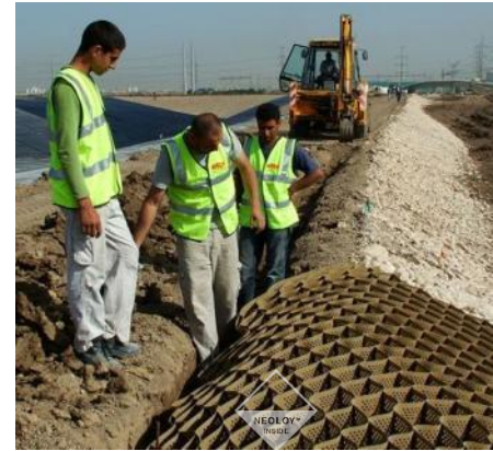
FIGURE 15. PLACING SECTION ON ANCHORS AT CREST
