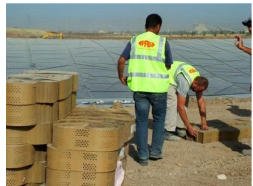
FIGURE 3. OFF-LOADING SECTIONS ON-SITE
