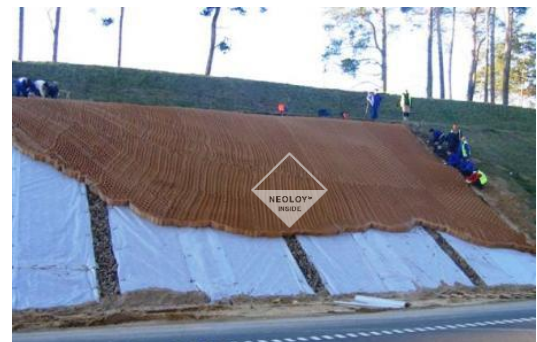
FIGURE 17. EXPANDING SECTIONS DOWNSLOPE
