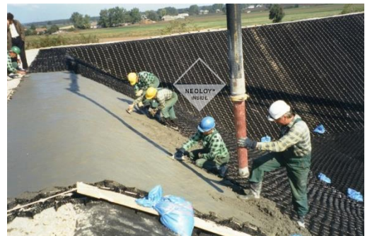
FIGURE 20. POURING AND SPREADING CONCRETE INFILL
