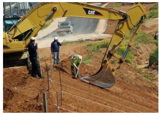
FIGURE 4. CLEAR AND SHAPE SLOPE
