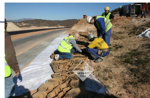
FIGURE 14. FASTENING SECTIONS FACE TO FACE
