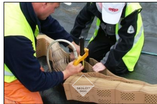
FIGURE 13. FASTENING END TO END
