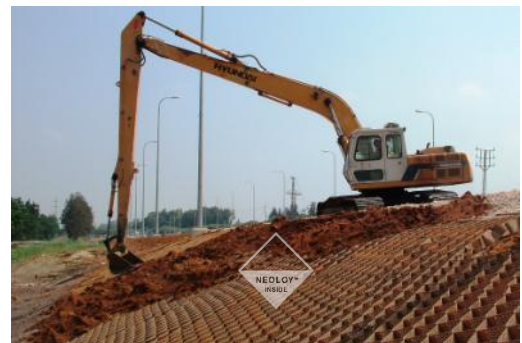
FIGURE 18. SOIL INFILL DOWNSLOPE BY EXCAVATOR
