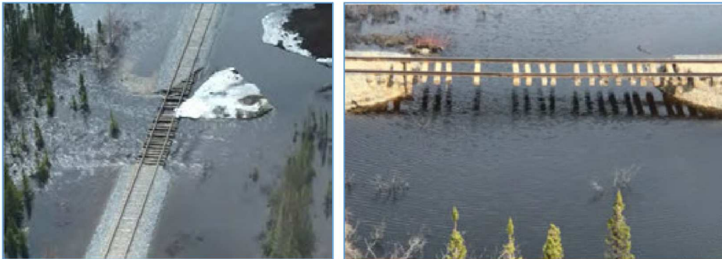
Figure 2. The railway line during the flood in 2017, aerial view. (Global News, 2017)
