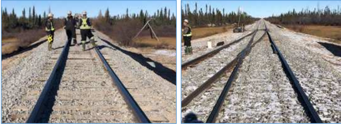
Figure 8. Completed rail re-installation at MP 427 and near switch at MP 414
