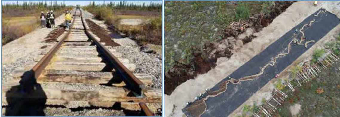
Figure 5. The track removal for the repair works
