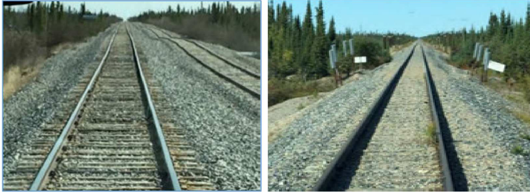
Figure 1. The condition of railway line in May 2016.
