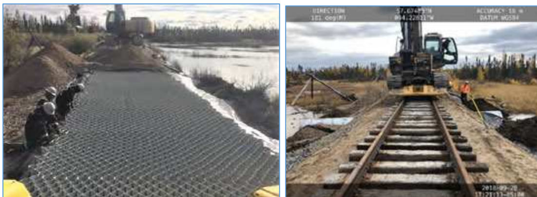
Figure 7. Geocell for sub-ballast reinforcement and section ready for ballast fill
