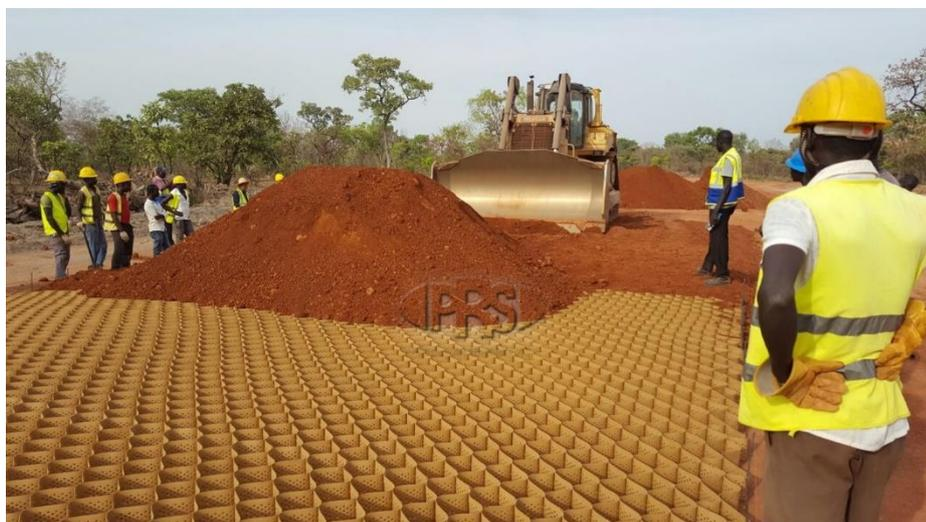
**Fig. 4.** Installation and infill of Neoloy Tough Cell on rural feeder road project
