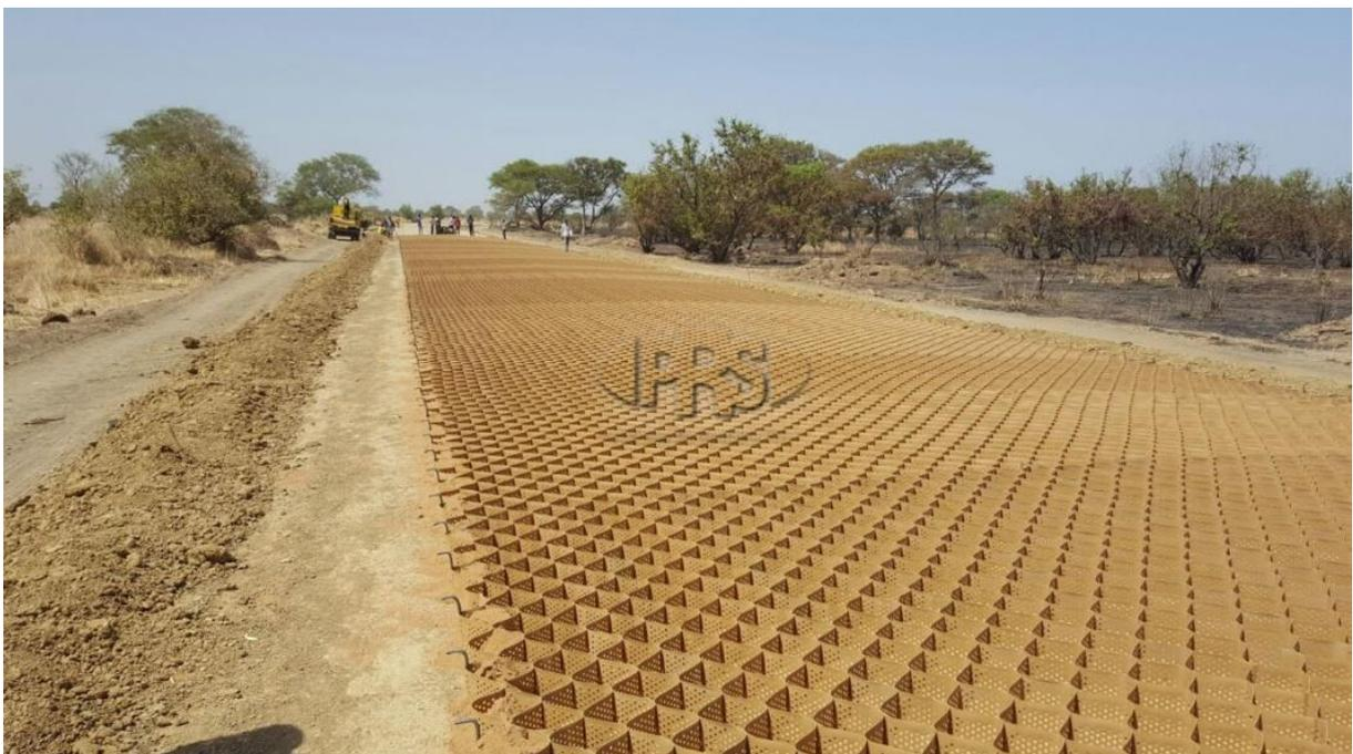
Fig. 1. Installation of Neoloy Tough Cell on Rural Feeder Road Project, UN
